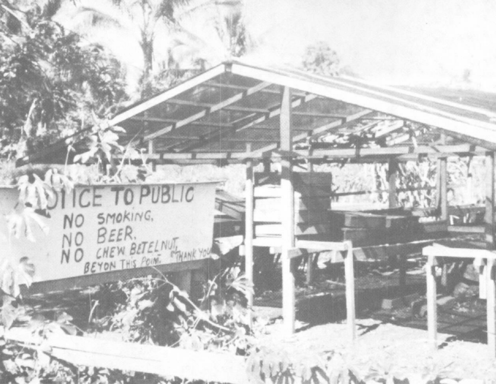
Development project outside of Honiara Courtesy Steven R. Pruett
